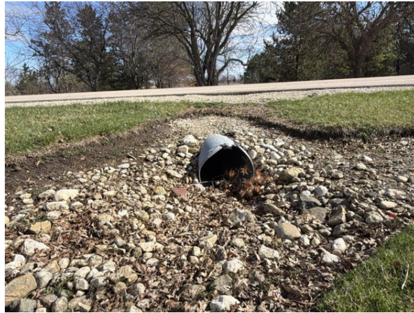
Photo 2: Culvert under Norris Road, facing northeast.
